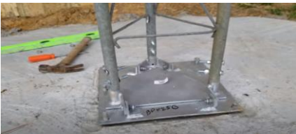
Machine Foundation Fixing
