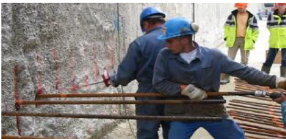
Rebar & Anchor Fixing on Bridge
