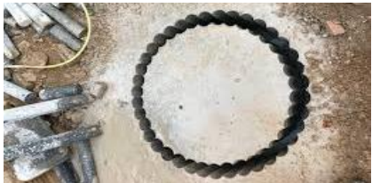
Stitch Coring for Large Opening
