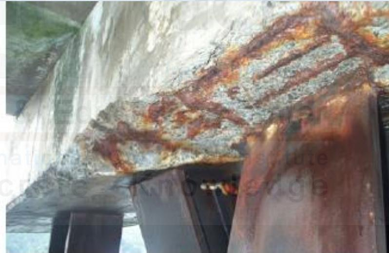
Figure 2. Typical corrosion damage
